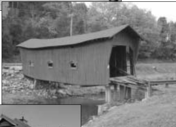
The Bible Covered Bridge, Greene County
