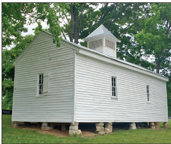
The 1850s carriage house at Clover Bottom was rescued from severely deteriorated condition, as shown by these “before and after” photos. The cupola was restored based on an 1898 photo found in the Price collection, profiled in the June, 2015 issue.
