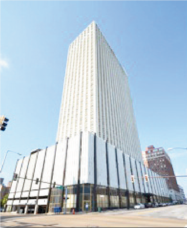
One Hundred North Main Building
