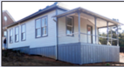
Clinic After Restoration
