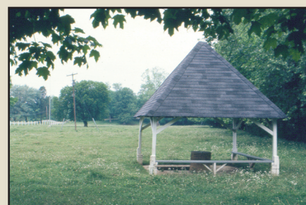
Figure 2 Salt Lick Gazebo today with concrete and metal pipe configuration.
