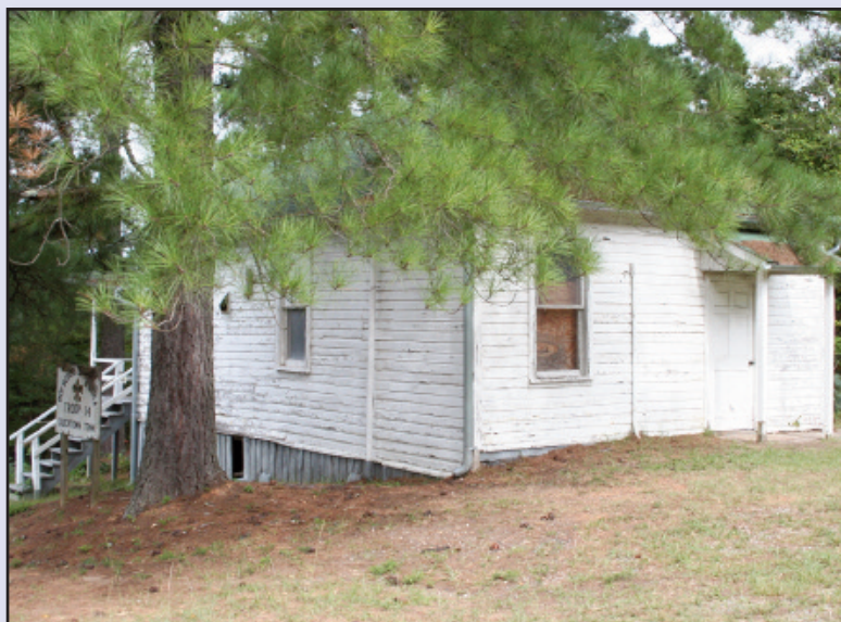
Before the Clinic restoration
