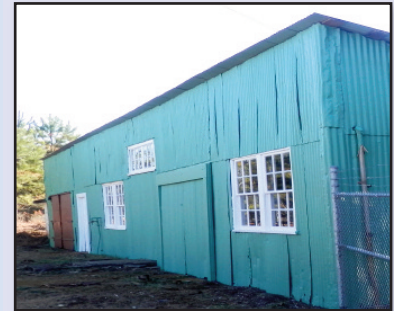
Plate Shop exterior after renovation
