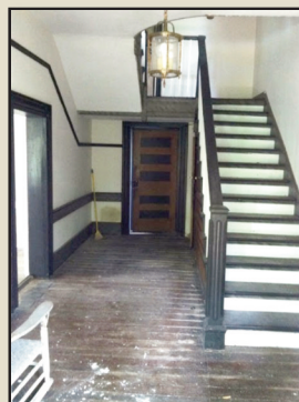
Figure 2. Byrd Brown House Stair hall
