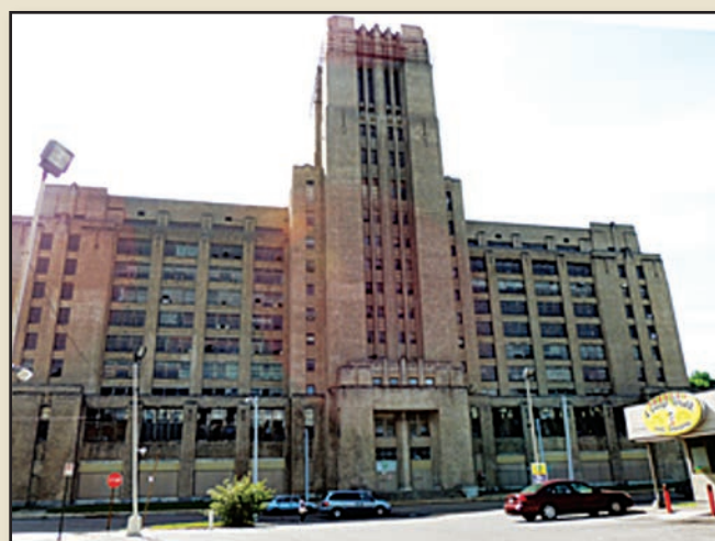
East elevation of Sears Crosstown
