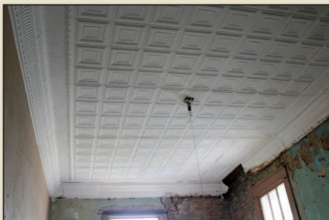
Detail of the pressed tin ceiling in the President's Office of the Red Boiling Springs Bank.
