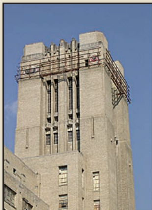
View of the tower. The scaffolding attached to the top was installed c. 1941 to hold large neon letters that spelled "Sears" on three of four sides
