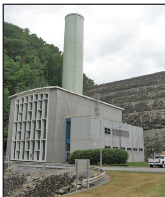
South Holston Dam, powerhouse, and surge tank.
