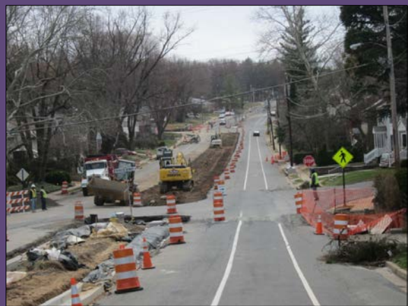
Photograph of roadway under construction for a green streets project in Arlington, Virginia. Project includes pedestrian intersection improvements and the creation of a bio-retention swale in the median. This project is part of the county's Neighborhood Conservation Program which directly engages citizens in identifying project scope and needs within their neighborhoods and prioritizing projects annually.
