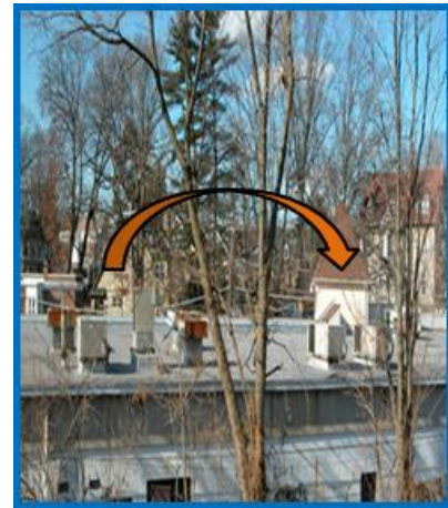
Air exhaust from a drycleaner with harmful chemicals next to air intake at a child care facility.
