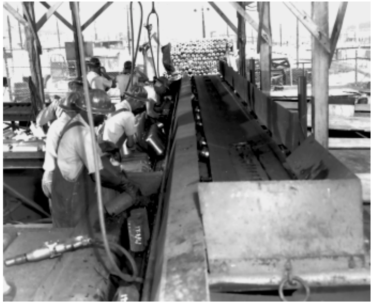
Workers at the Y-12 mercury dumping shed. Pipelines carried mercury to the buildings that housed Colex operations.
