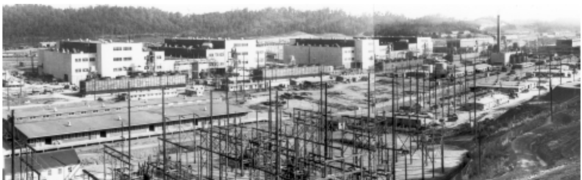
A 1945 view of a portion of the Y-12 Plant. The large buildings in the center housed devices called calutrons for electromagnetic enrichment of uranium during World War II. These same buildings were sites of lithium enrichment processing in the 1950s and 1960s that used large quantities of mercury.
