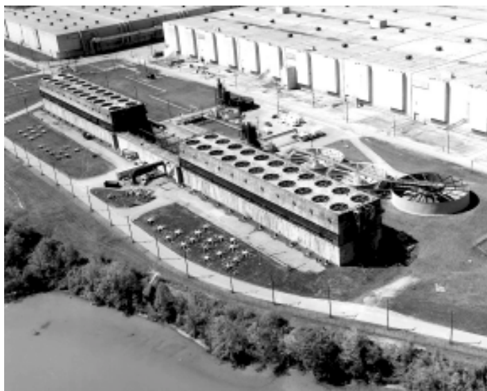
Hexavalent chromium was used as a corrosion inhibitor in the water that flowed through cooling towers such as these at the K-25 Site. Poplar Creek is at the lower left.
