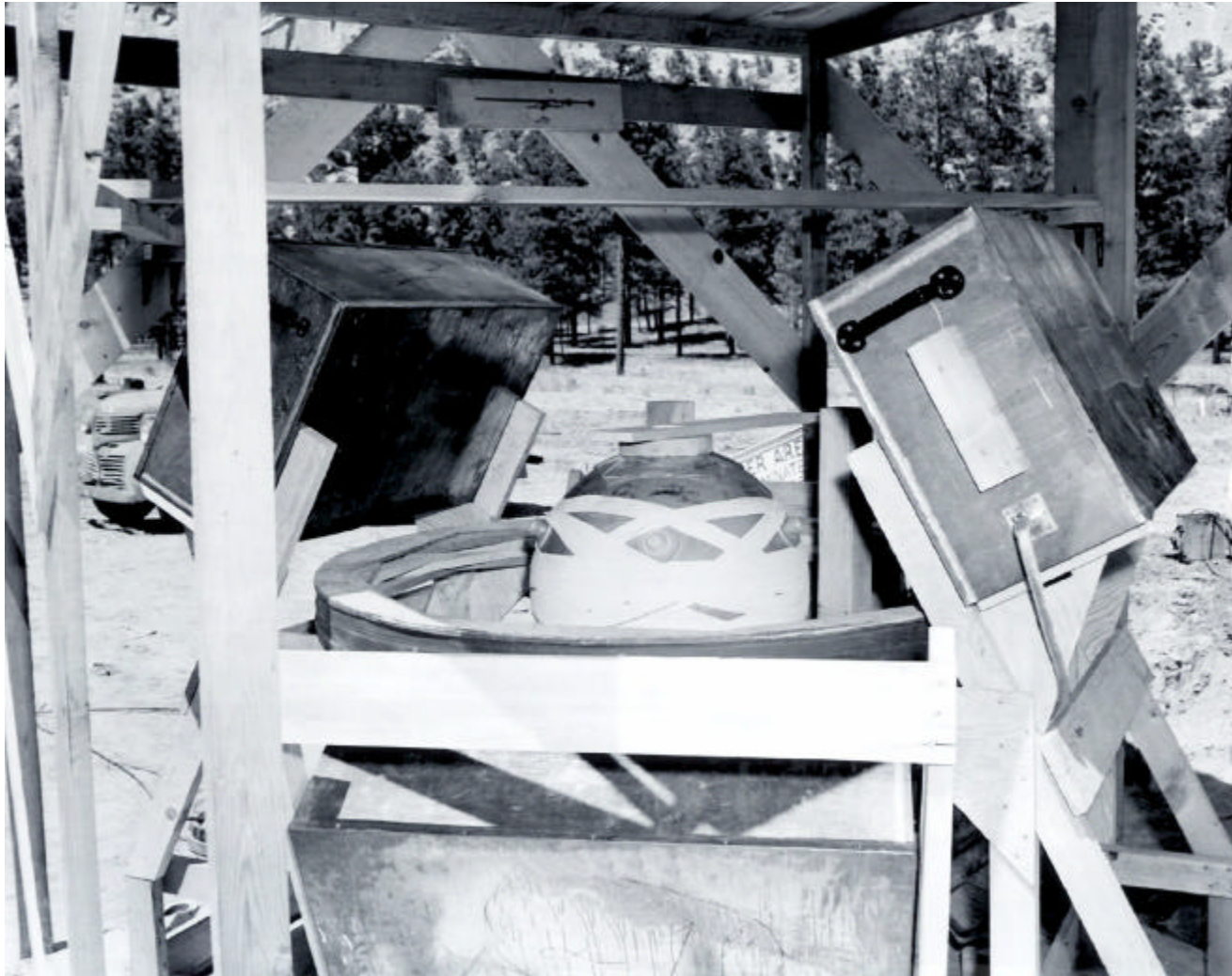
Photograph 1: Los Alamos Apparatus for Using RaLa to Test the Implosion Process
