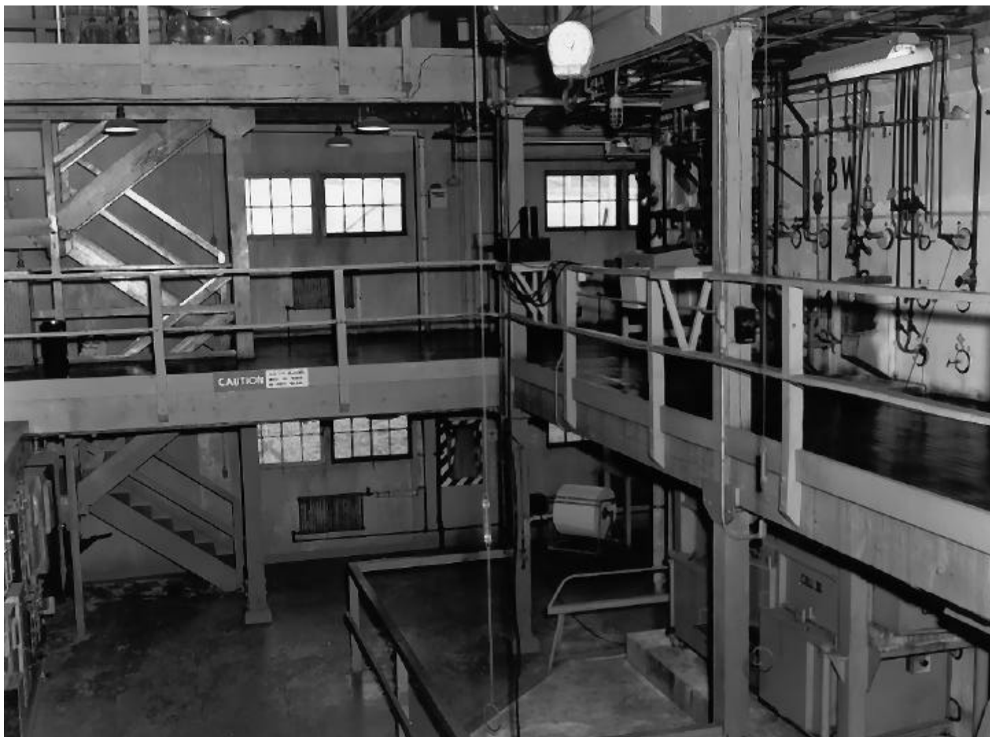
Photograph 3: Interior View of the Building 706-D RaLa Processing Facility
