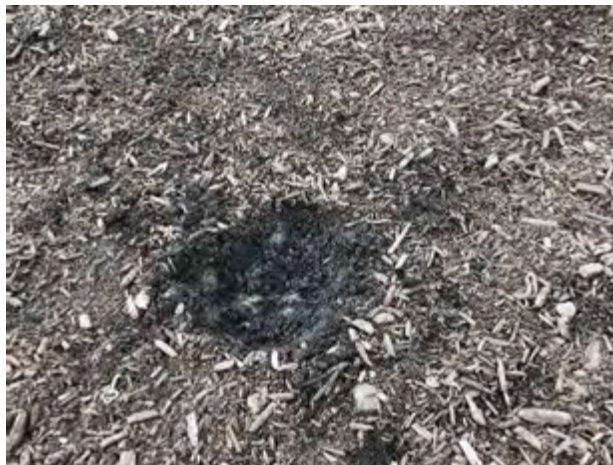
Photo 4: High traffic area, beneath the swing set located within the playground area in the northeast corner, where a soil/mulch mix was observed and the geotextile fabric was compromised (CLX-SL-PGIN-14)
