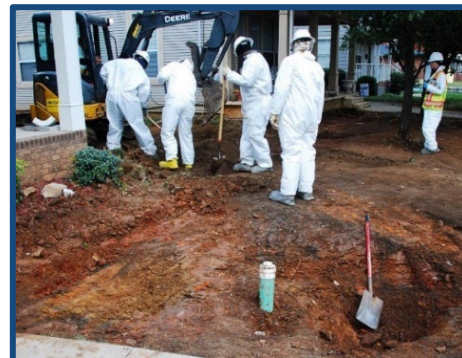
A yard in SSCL site during remediation.
