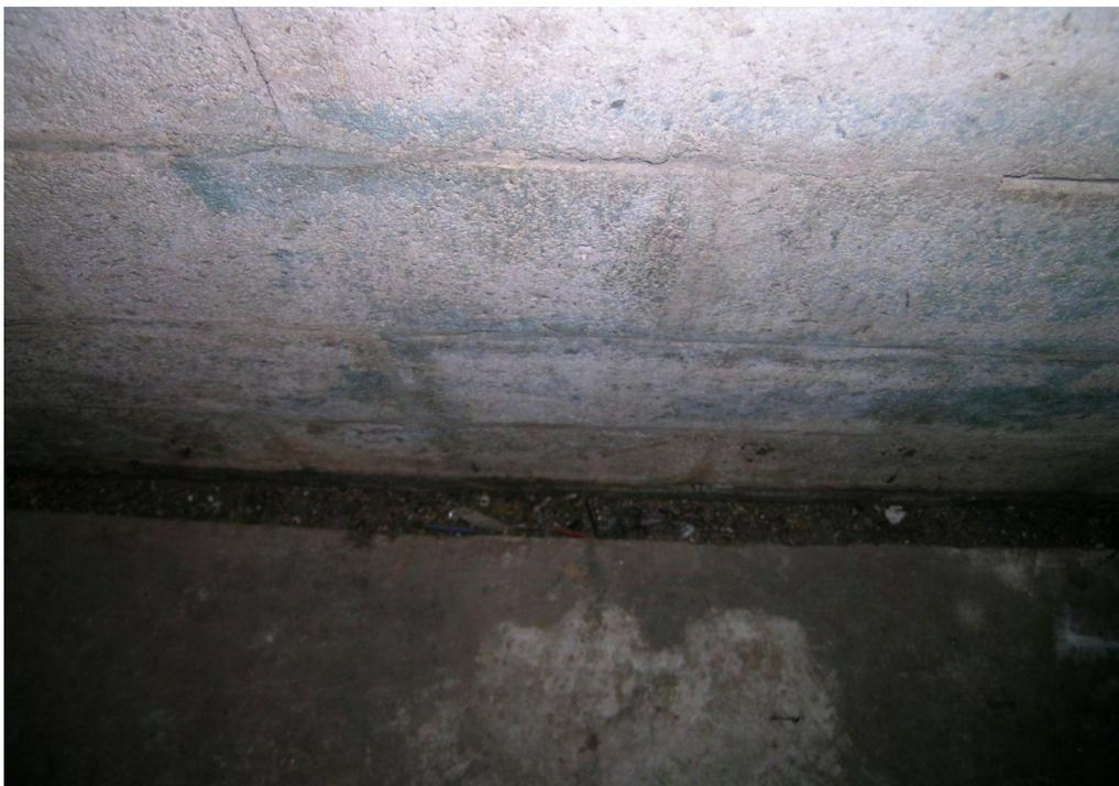
**Photo 4** - View of trench that drains water from the basement walls to the corner sumps in Home A. Water from the outside soils or from a high water table could contain chemicals which could lead to vapor intrusion in the home (Photo credit: TDH, 04/18/11).
