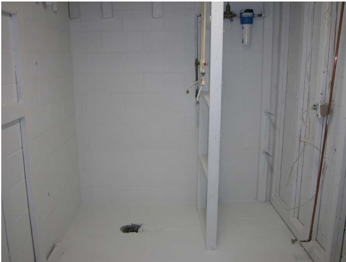
Figure 4. Basement bathroom after remediation
