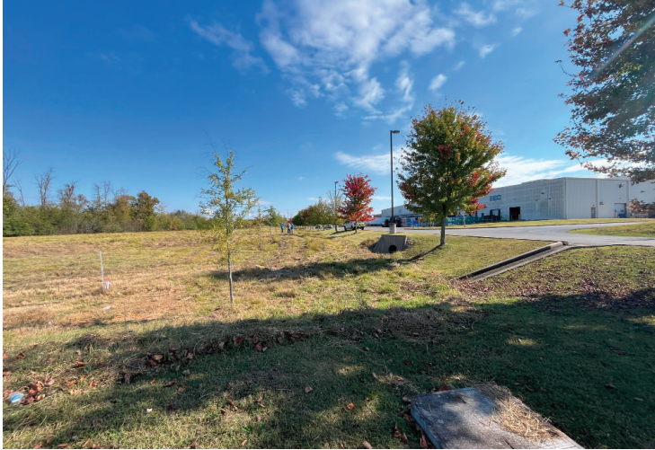
Existing site conditions at Rutherford County
