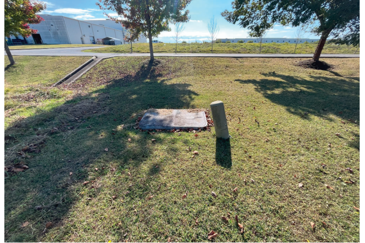
Existing site conditions at Rutherford County
