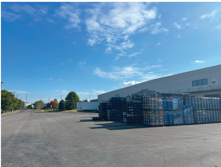
Existing site conditions at Rutherford County
