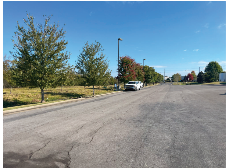
Existing site conditions at Rutherford County
