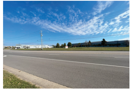
Existing site conditions at Rutherford County
