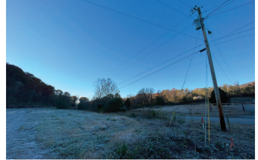
Existing site conditions at Anderson County
