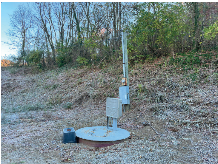
Existing site conditions at Anderson County
