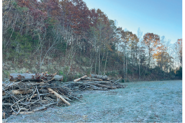
Existing site conditions at Anderson County
