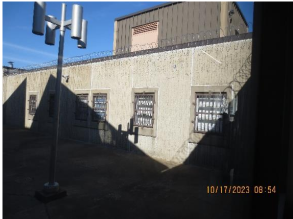
S3 - View to Courtyard
