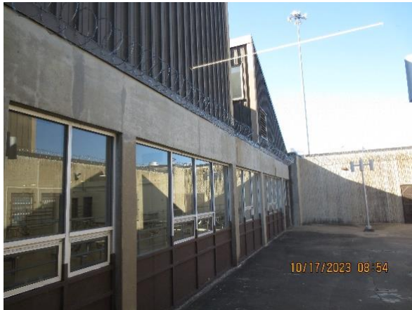
S1 - View to Courtyard
