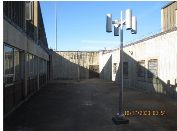
S2 - View to Courtyard
