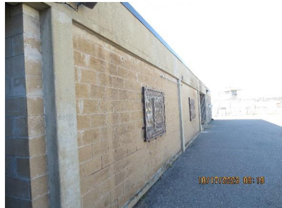
S4 - View to Infirmary Building
