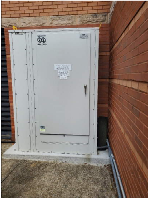
Photo B5: Existing 1200A Storm Switch
