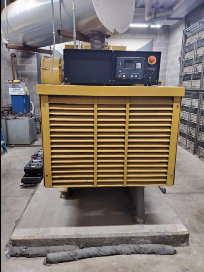
Photo B1: Main Hospital 750kW Generator
