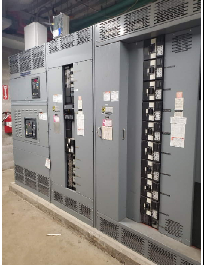
Photo B2: Main Hospital Main Switchboard
