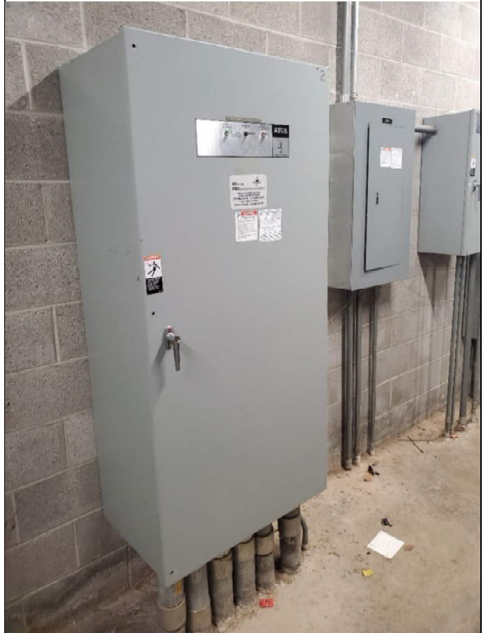
Photo B4: CRDP Transfer Switch
