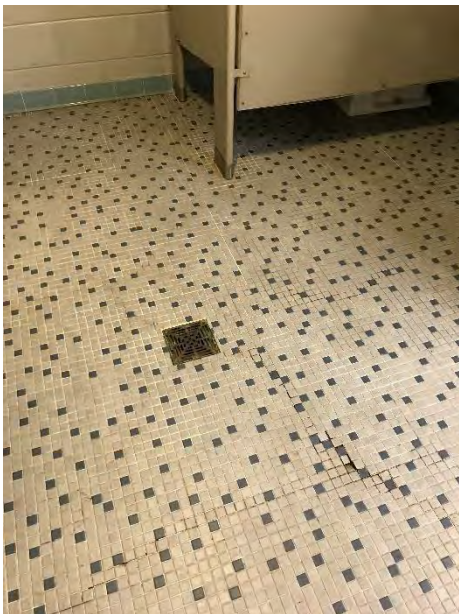
113) Second Floor Men's Room
