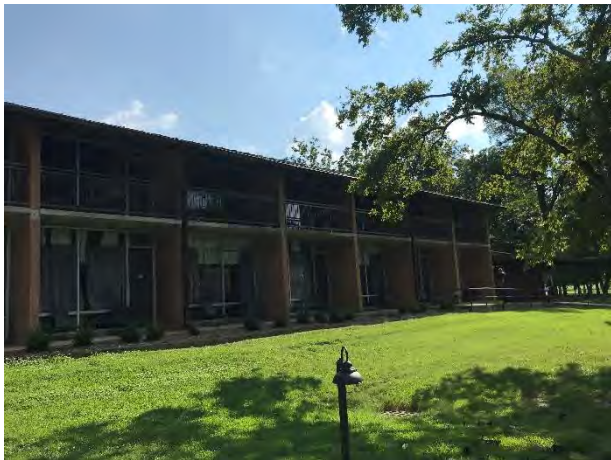
7) Lodge Exterior - View of north facing rooms on the west wing.
