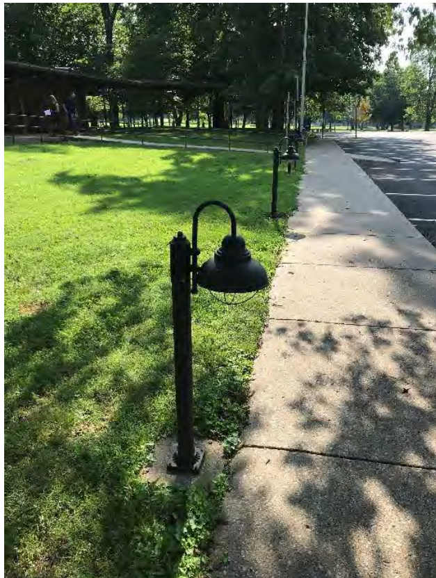
8) Lodge Exterior – Sidewalk along north parking lot looking west. Post lights have more than a 4” projection and are a possible ADA obstruction.
