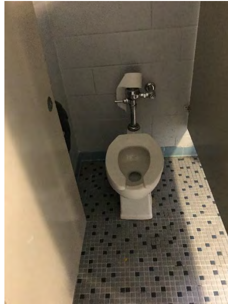
110) Second Floor Men's Room –
