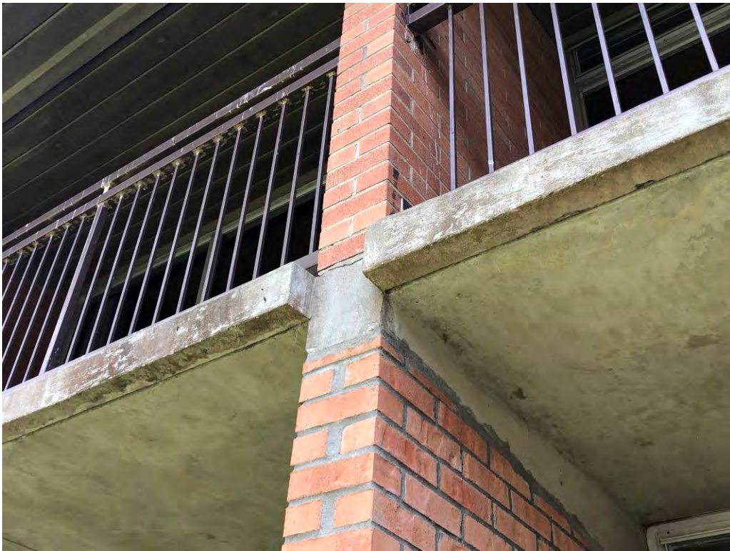
Photograph 4 – Second floor concrete balconies bearing on masonry walls.
