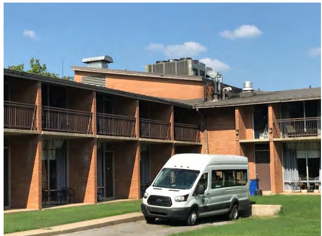
12) Lodge Exterior – Close up view from the southwest. Note location of linen delivery parking near the exterior door to the first floor housekeeping room.
