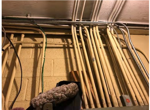
177) First Floor Janitor / Electrical
