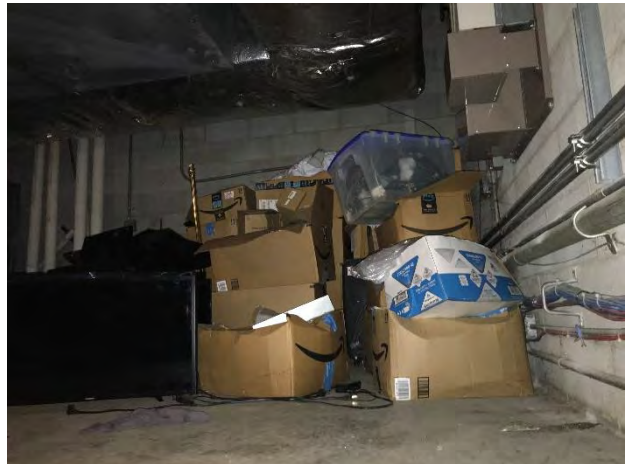
189) Second Floor Mechanical Room
