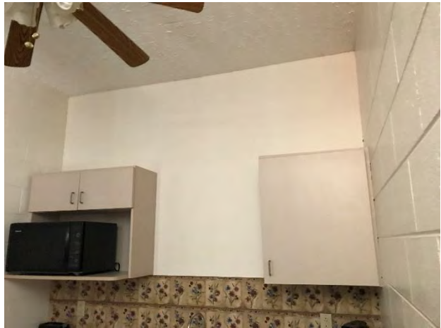
73) Guest Room 102 – View of Kitchenette
