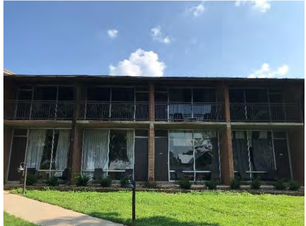
6) Lodge Exterior – View of north facing rooms on the west wing.
