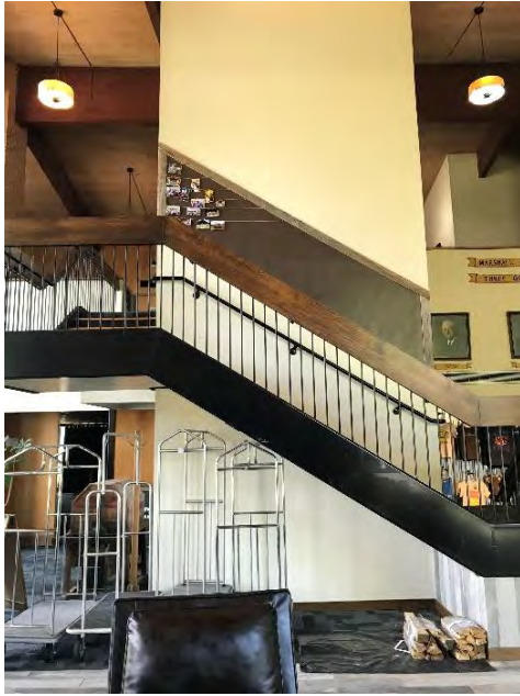
23) Lobby – View of open stair to the second floor. The original stair was re-configured when the elevator was added in the late 1990's.
