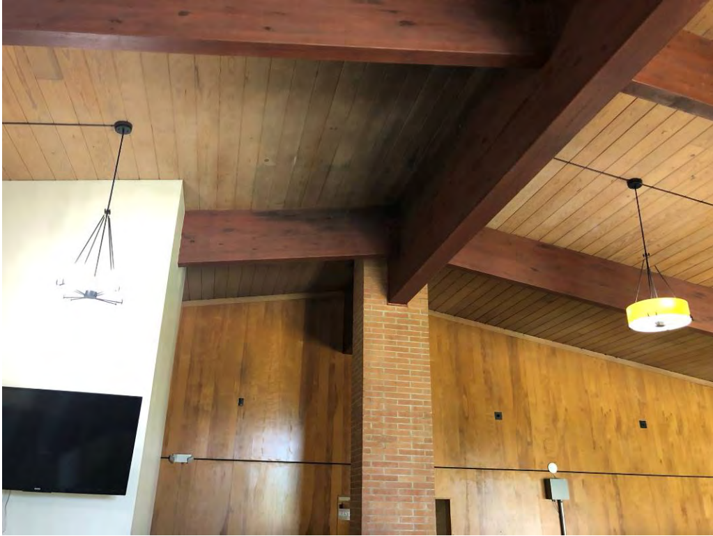
Photograph 9 – Roof framing at lodge lobby.
