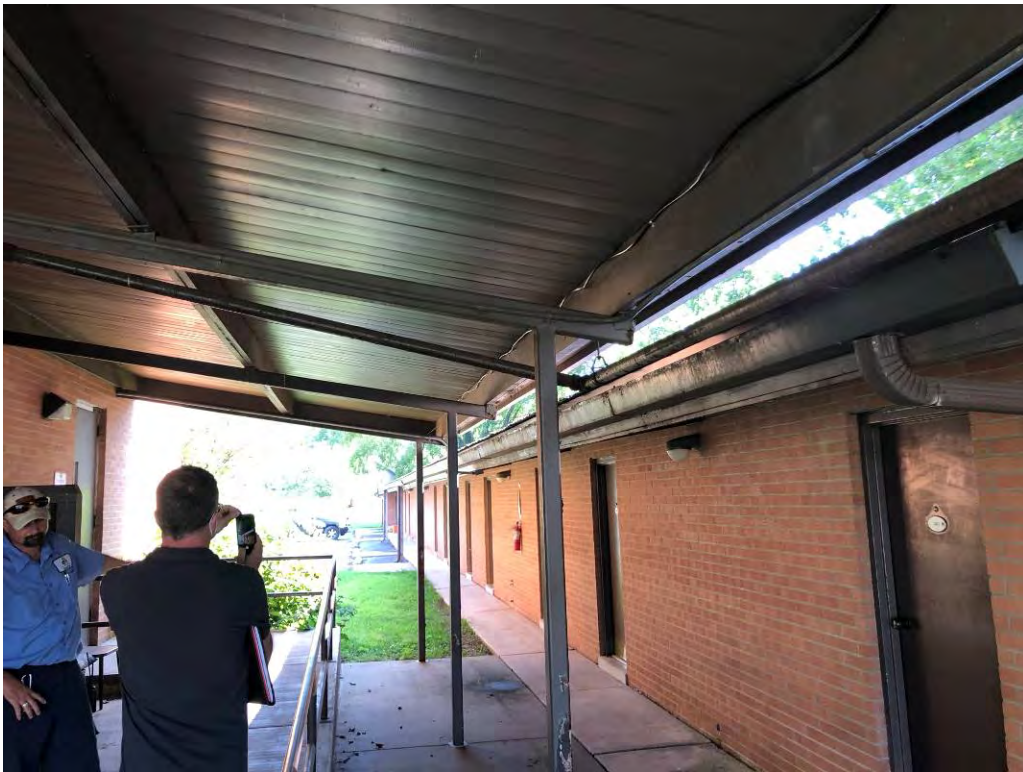
Photograph 14 – Canopy between lodge and motel.
