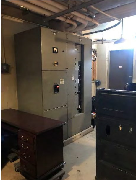
98) First Floor Housekeeping -
