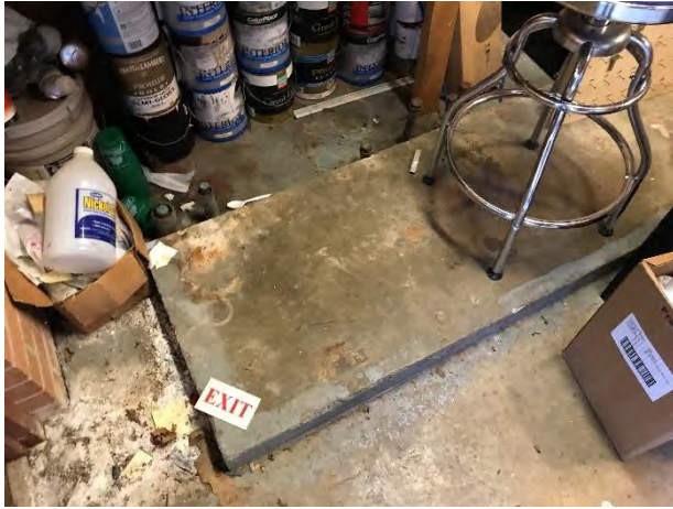
221) Motor Court Mechanical Room
