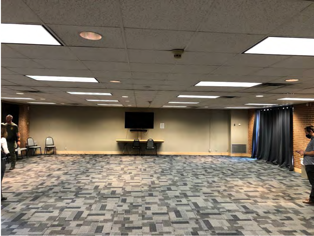
Photograph 13 – Lodge conference room. Structural steel beams and concrete slab structure above.
