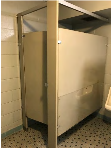
109) Second Floor Men's Room –
