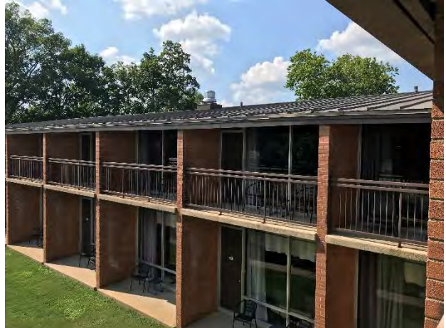
14) Lodge Exterior - View looking at the south side of the west guestroom wing.
