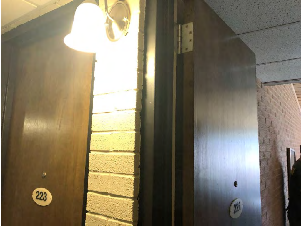
Photograph 11 – Load-bearing walls at second floor corridor.
