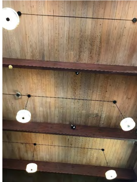
22) Lobby – View of wood deck ceiling, beams, and lighting.
