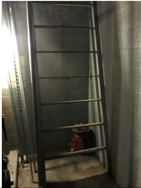
188) Second Floor Mechanical Room
