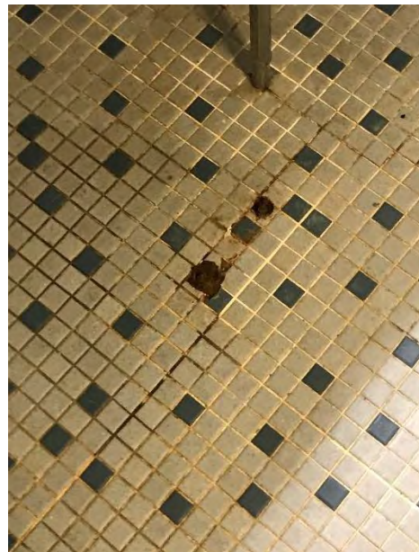
114) Second Floor Men's Room -
