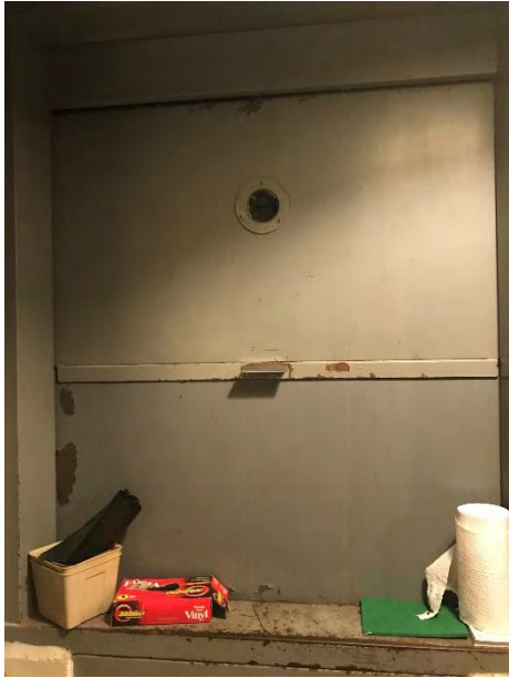
96) First Floor Housekeeping - .
