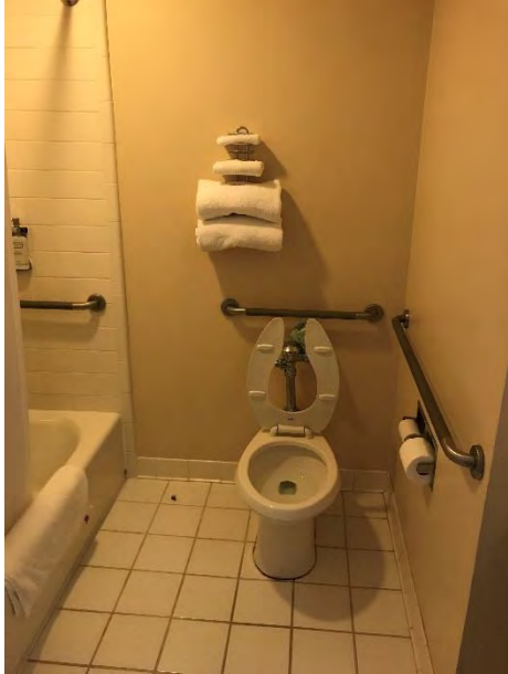
74) Guest Room 102 – View of bathroom and grab bars at toilet.
