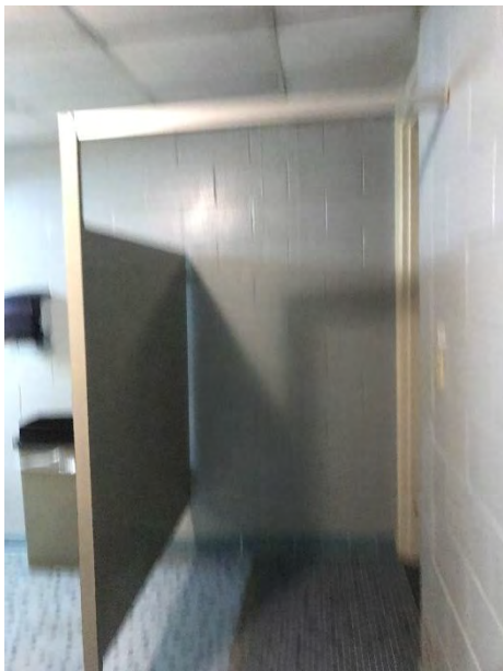
69) First Floor Men's Room –
