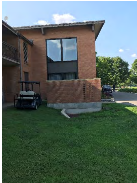
18) Lodge Exterior – View along the southeast façade looking north.
