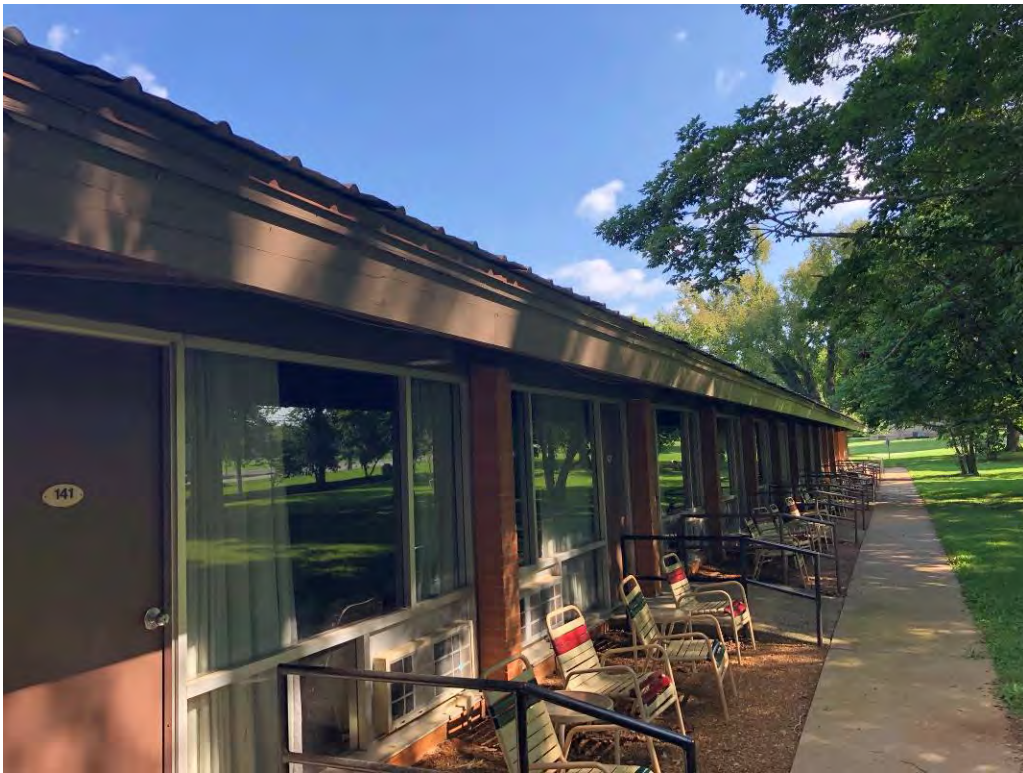
Photograph 16 – Exterior view of motel from west side.
