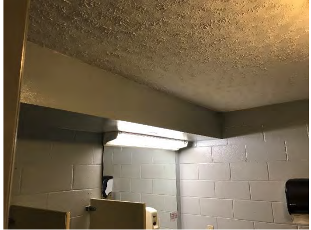
108) Second Floor Men's Room –
