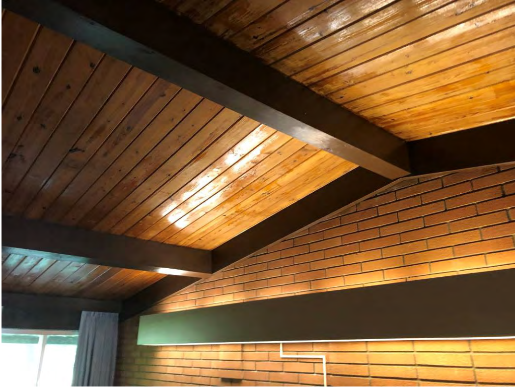
Photograph 17 – Typical roof structure in motel room.
