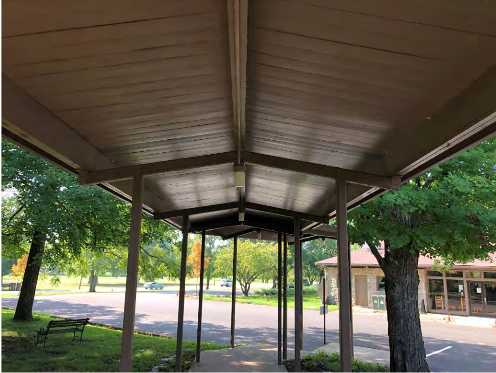
Photograph 15 – Exterior covered walkway.
