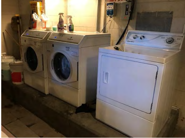
92) First Floor Housekeeping - recommended.
