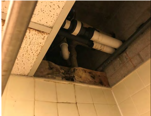
56) Board Room Restroom -
