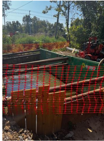
Trench box with pumps at Mt. Juliet site
