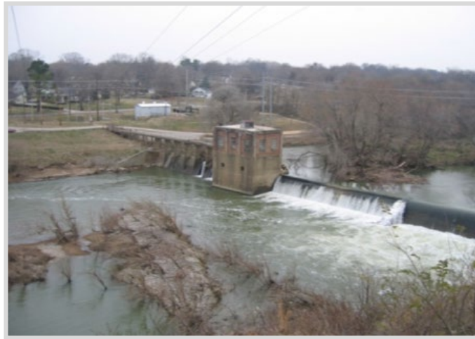
Figure 4 Columbia Dam on Riverside Drive
