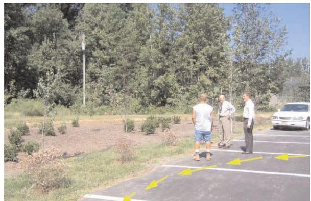
*Some site runoff bypasses bioretention because of inadequate slope of filter strip.*
