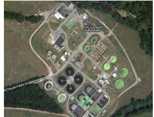
Franklin Water Reclamation Plant
