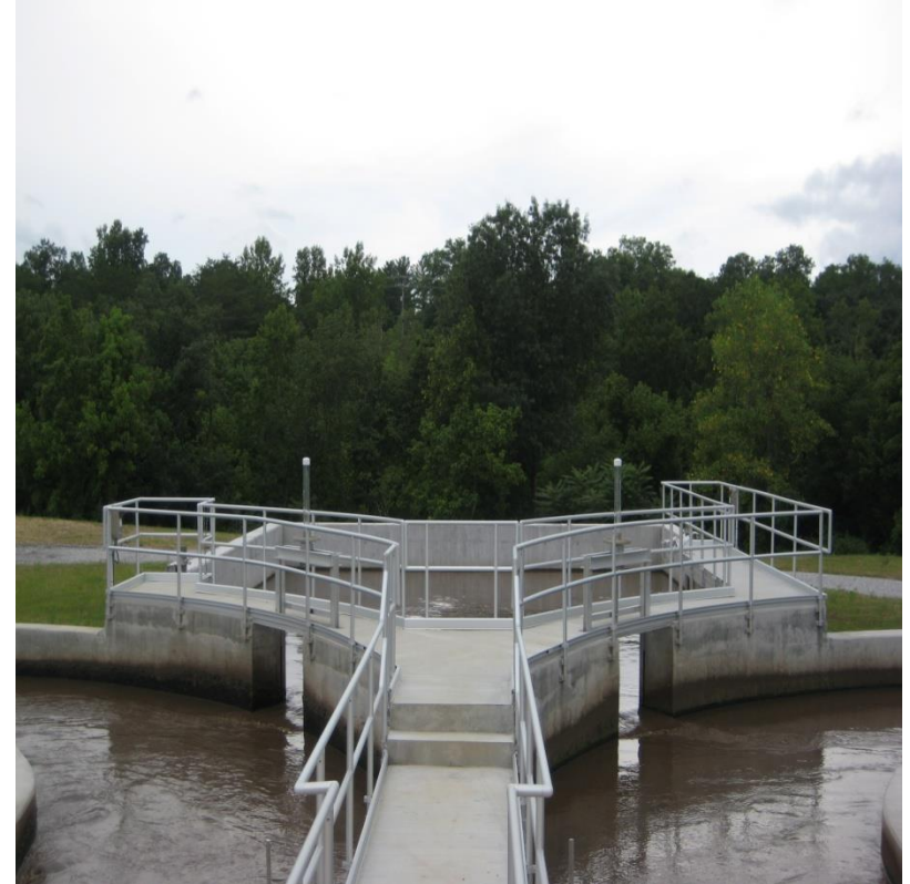
Anaerobic Zone
