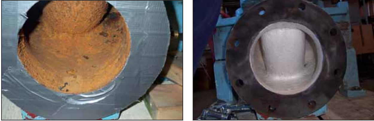
Figure 4.12 MCWA pump interior before (left) and after (right) sandblasting and coating
