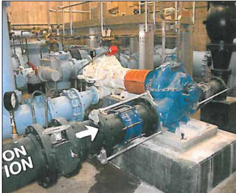
Figure 4.9 Recirculation pump
