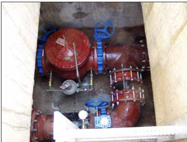
Figure 4.14 Altitude valve at Luzerne Road Tank
