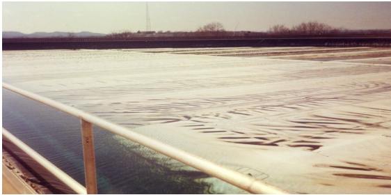
This is an old open-topped (8 th Ave) reservoir that has been converted with a liner-cover
