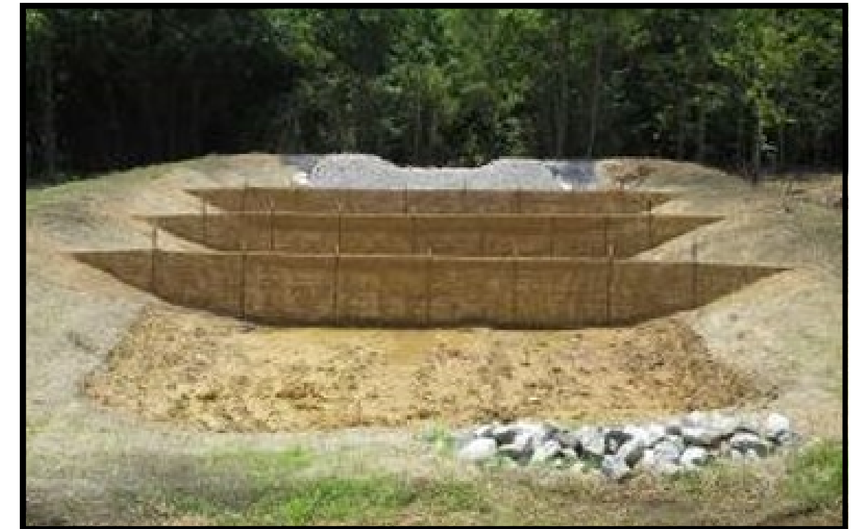
Example of a sediment trap included in the TNEPSC Handbook.
