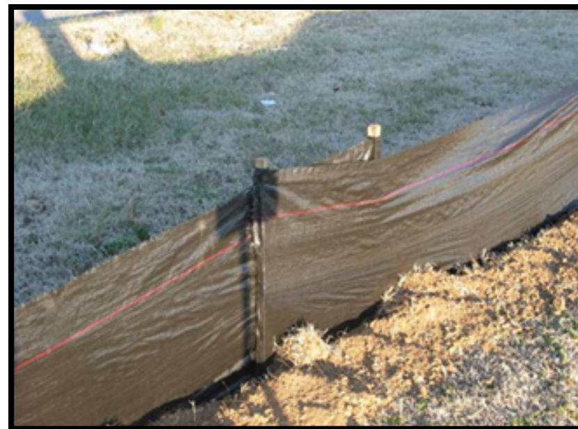
Example of silt fence included in the TNEPSC Handbook.
