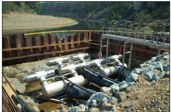
Figure 9. Possible intake screen configuration (photo courtesy of Johnson Screens)
