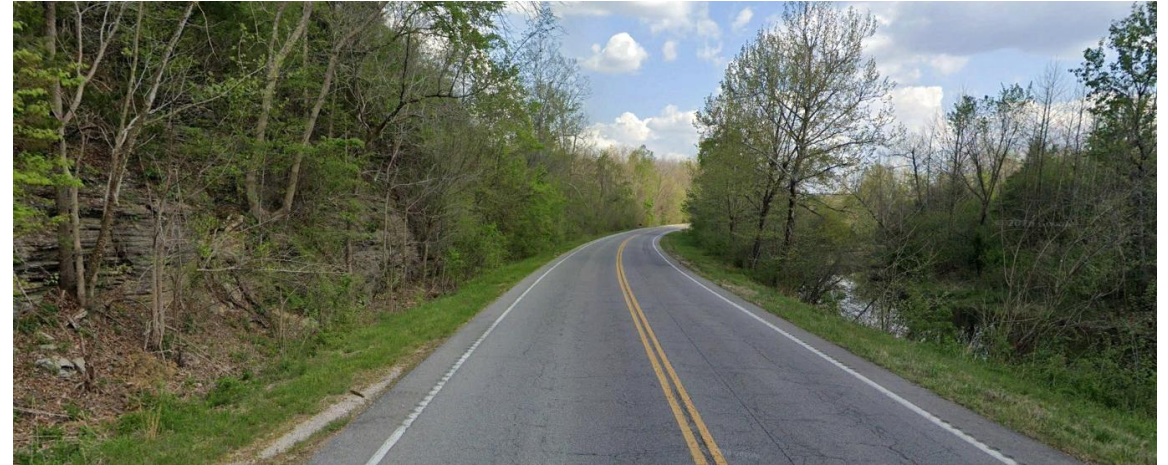
Two-lane rural corridor with steep cut slope limiting ROW width
