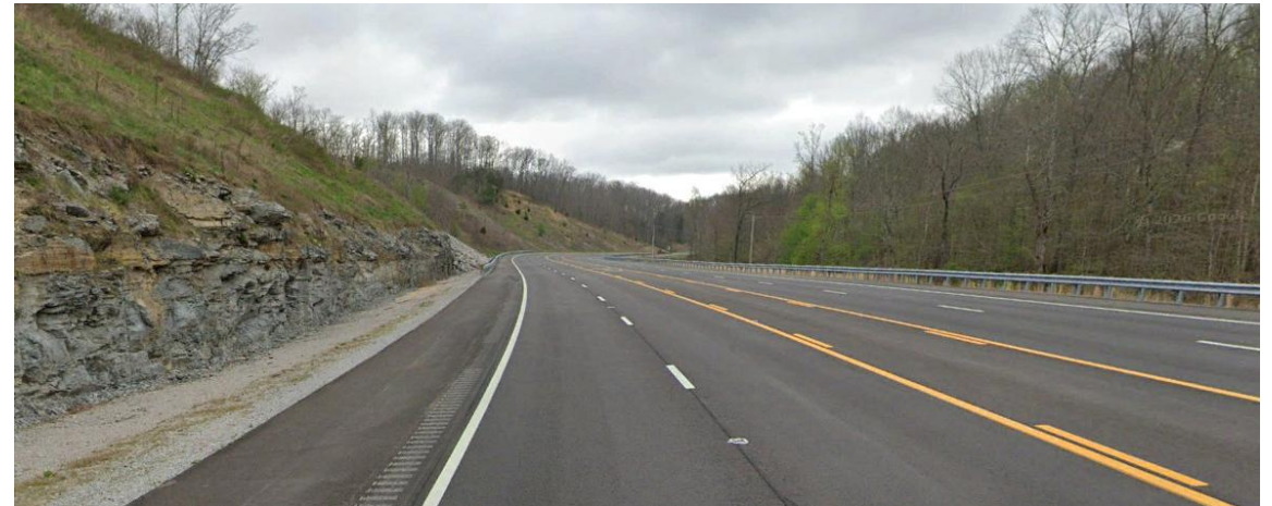
Recently widened section with rock cut through the ridge
