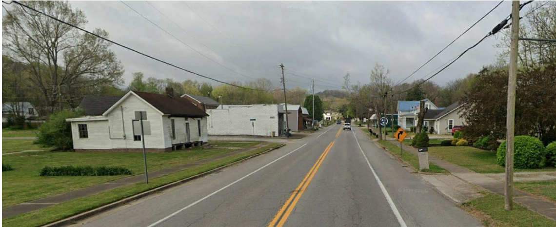
Residential frontage constraining ROW along the tight corridor through Hampshire
