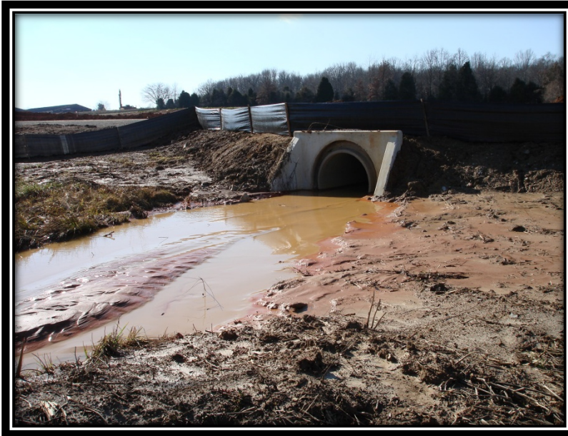
Poor stabilization during construction. Photo provided by Jimmy Smith, NRS.
