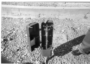
Acceptable sampling station at foot of water tank
