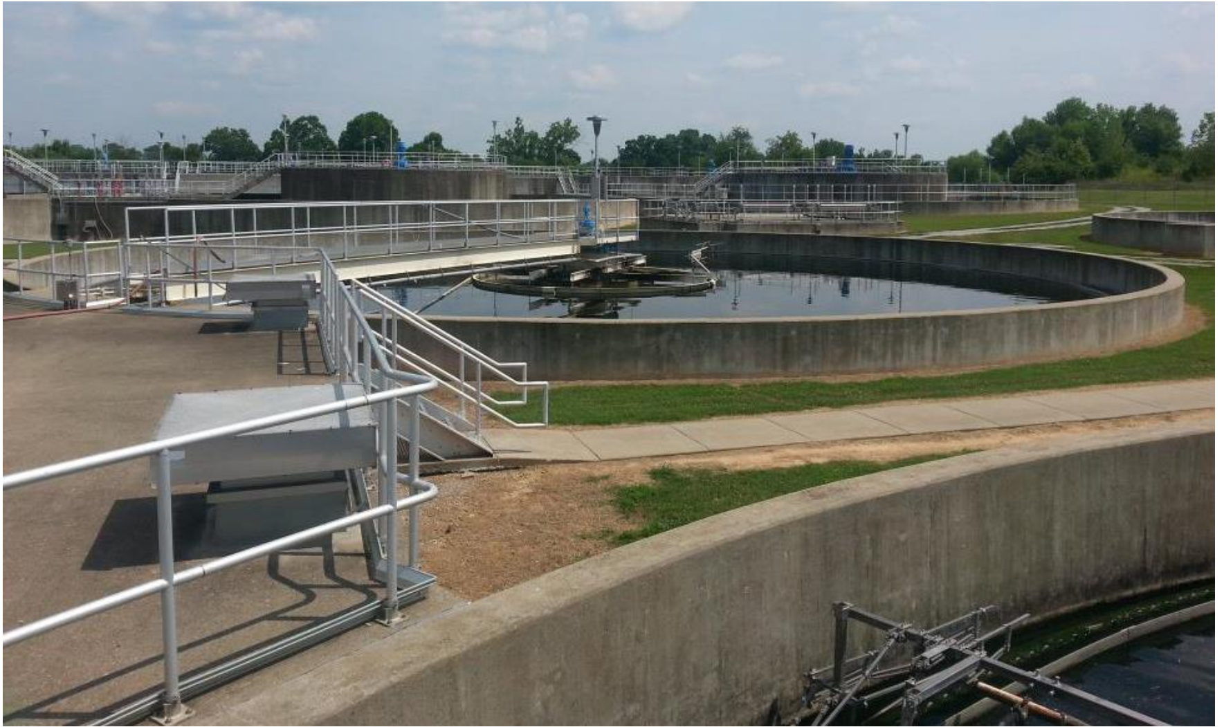
City of Franklin Wastewater Treatment Plant
