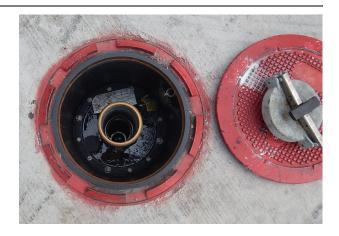
Please remember to empty fuel/water/debris from your spill bucket and manage wastes properly.
