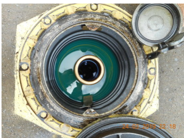
Diesel in spill bucket
