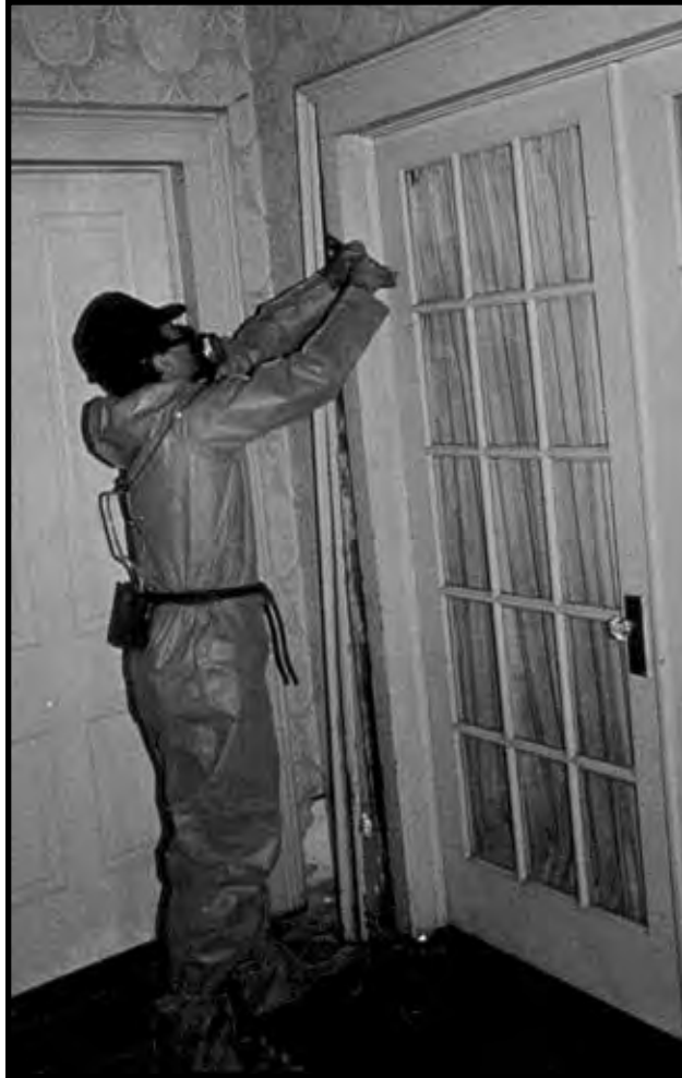
Figure 12.3a Remove and Replace Trim (interior).
