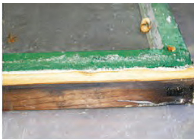
FIGURE 11.11 Wet plane edges of sash to fit new jamb liners.
