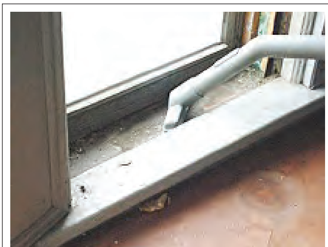
FIGURE 11.5 Prepare the worksite and pre-clean the window.
