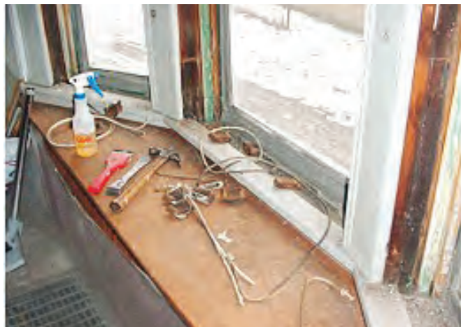
FIGURE 11.9 Window after removal of sash weights.
