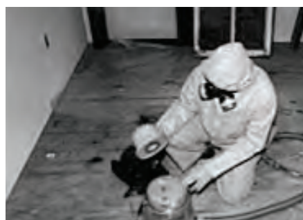
f) Remove & Replace HEPA Filter Assembly.
