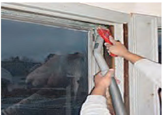
FIGURE 11.12 Vacuum window again.
