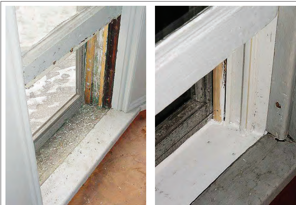
FIGURE 11.3 Window before and after friction treatment.
