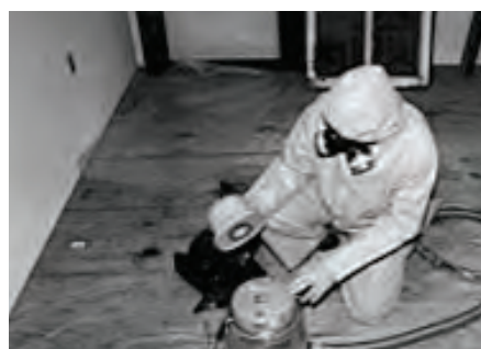
c) Remove Bag with a Plastic Sheet Underneath
