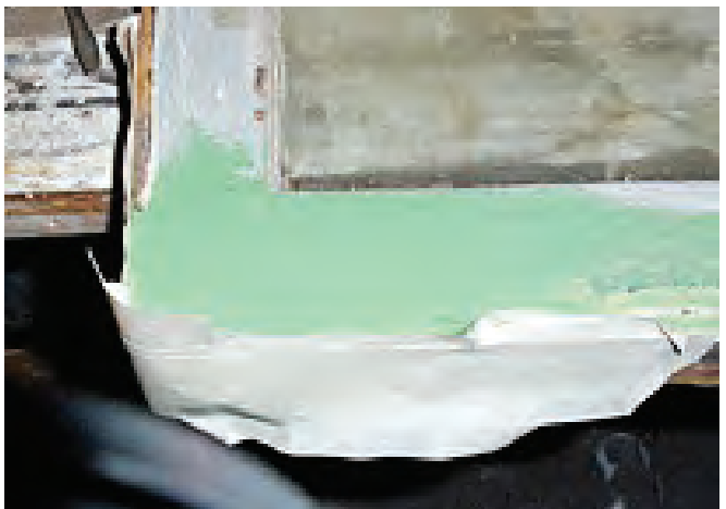
FIGURE 11.10 Rebuild damaged sash with filler or putty.
