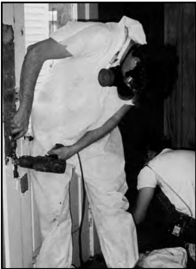
Figure 12.15 Heat Guns Operating Below 1,100 °F Are Useful for Limited Areas.
