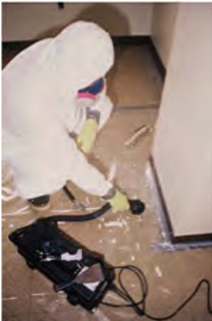
FIGURE 14.8 Vacuuming the floor containment.
