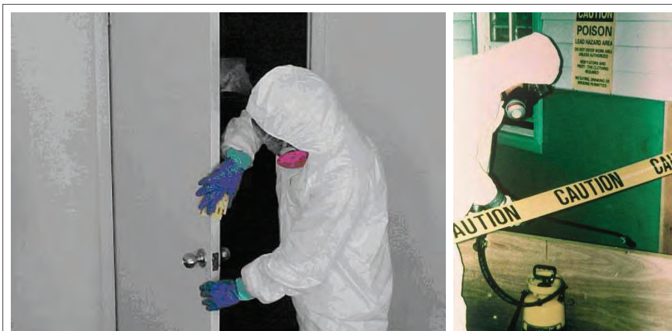
FIGURE 11.15 Stabilizing paint on doors: Wet planing (left) and wet sanding (right) deteriorated paint can create significant amounts of dust.
