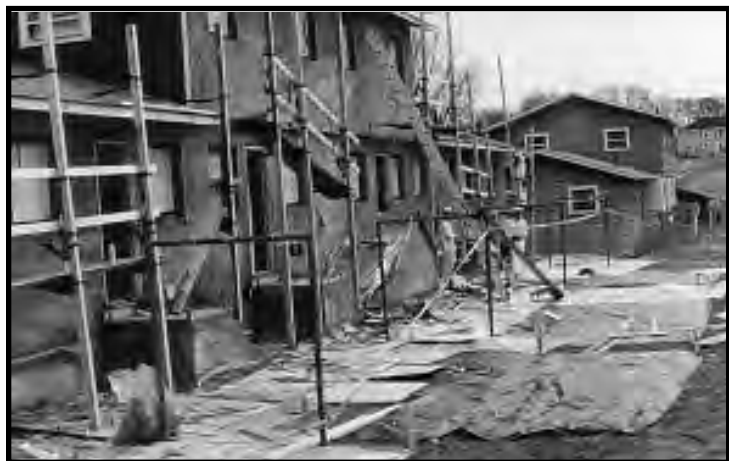
Figure 12.6 Exterior Siding Removal and Replacement.
