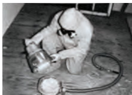
a) Remove the HEPA Vacuum Filters and Disassemble the Vacuum
