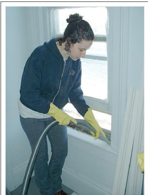
FIGURE 8.17 Pre-cleaning window with HEPA vacuum.
