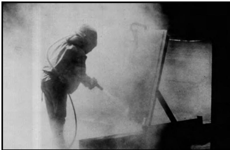
Figure 12.13 Traditional Abrasive Blasting Is Prohibited (note the visible dust surrounding the worker).
