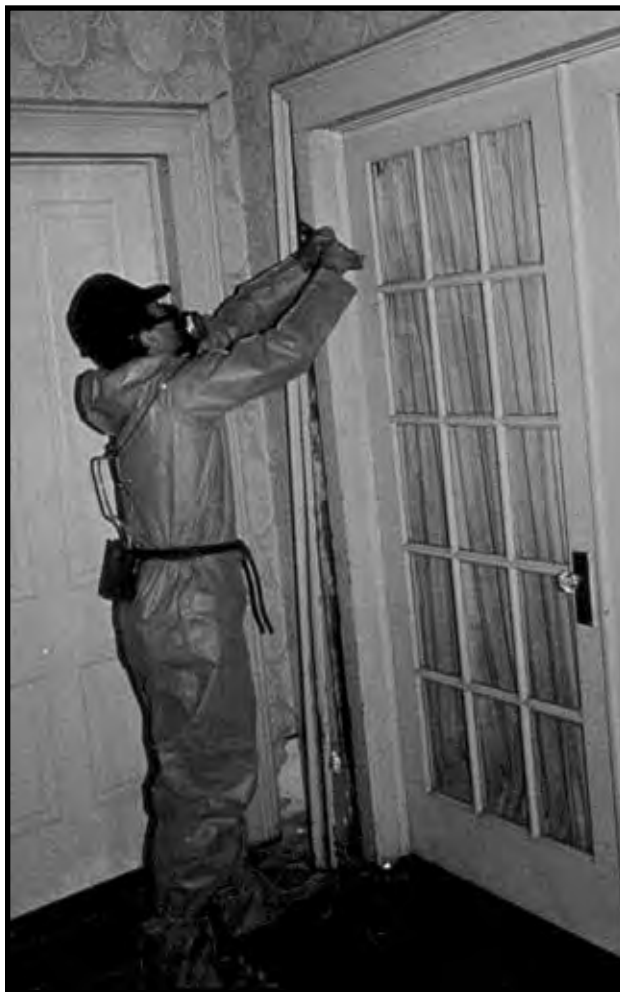
Figure 12.3a Remove and Replace Trim (interior).
