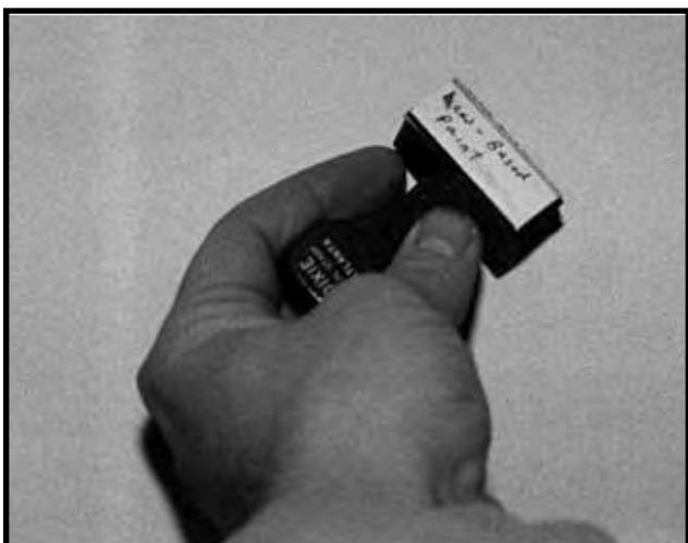
Figure 12.8a Label Surfaces With a Stamp Before Enclosure.
