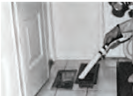
a. Vacuum and remove register covers;
