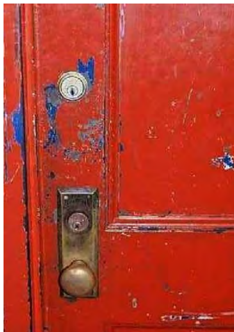
FIGURE 1.3 Paint deterioration.
