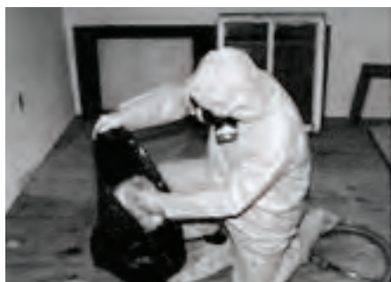
d) Tape Vacuum Bag Closed and Put Inside Plastic Trash Bag
