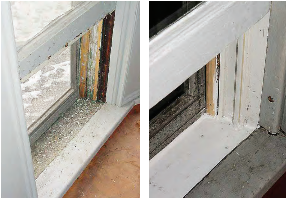
FIGURE 11.3 Window before and after friction treatment.
