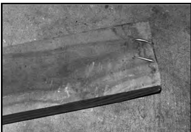
Figure 12.2 Bend Back All Nails on Removed Components.
