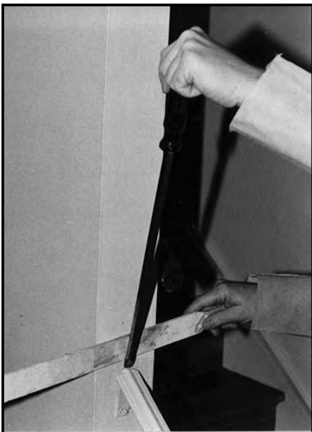
Figure 12.1 Use a Pry Point Pad To Minimize Damage to Adjoining Surfaces During Component Removal.
