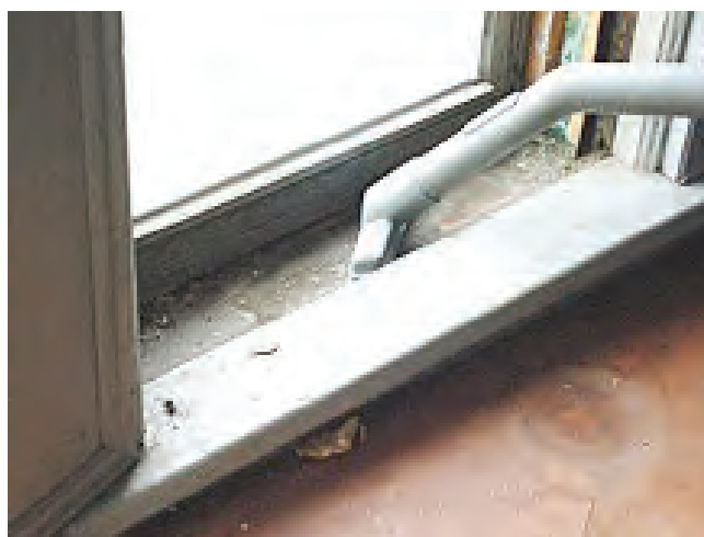
FIGURE 11.5 Prepare the worksite and pre-clean the window.
