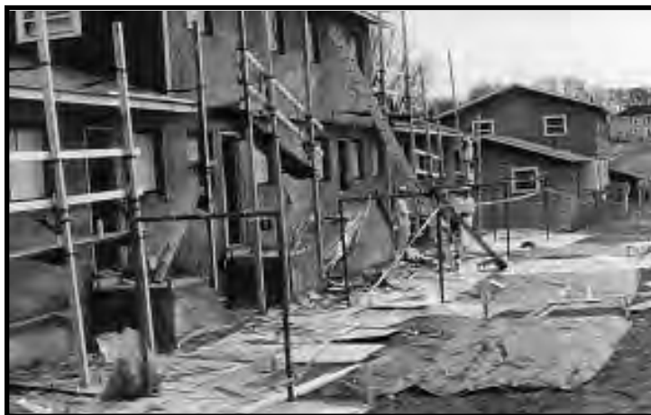
Figure 12.6 Exterior Siding Removal and Replacement.
