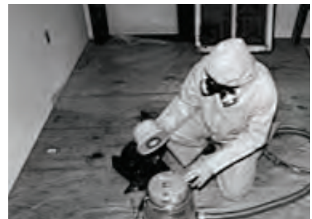
c) Remove Bag with a Plastic Sheet Underneath
