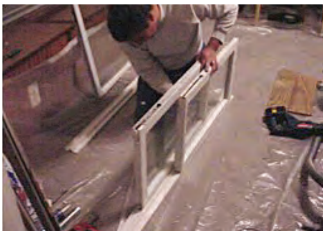
Figure 11.13 Fit sashes into jamb liners.
