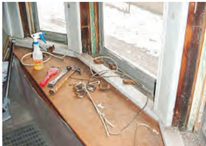
FIGURE 11.9 Window after removal of sash weights.
