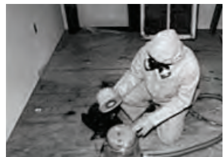
f) Remove & Replace HEPA Filter Assembly.
