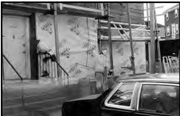
Figure 12.10a Use of Tyvek on Building Exteriors Prior to Enclosure.
