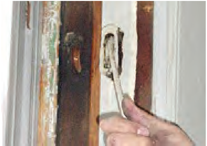
FIGURE 11.8 Remove sash controls/weights.
