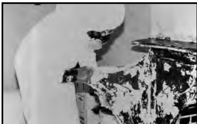
Figure 12.23a Neutralize Surfaces When Using Caustic Paint Removers.
