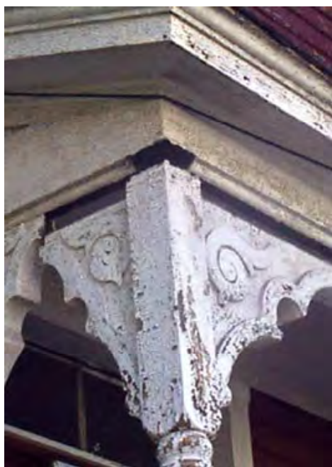
FIGURE 1.2 Deteriorated residential paint on house trim.
