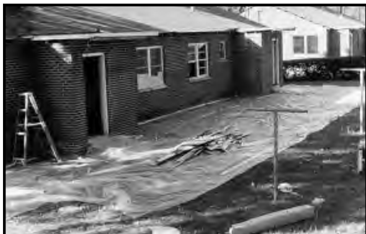
Figure 12.7a Line Walking Surfaces With Plastic.
