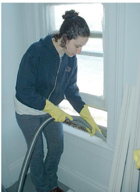
FIGURE 8.17 Pre-cleaning window with HEPA vacuum.
