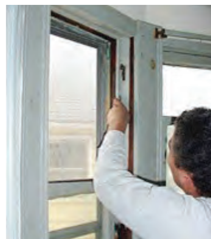
FIGURE 11.6 Remove parting Aboard.
