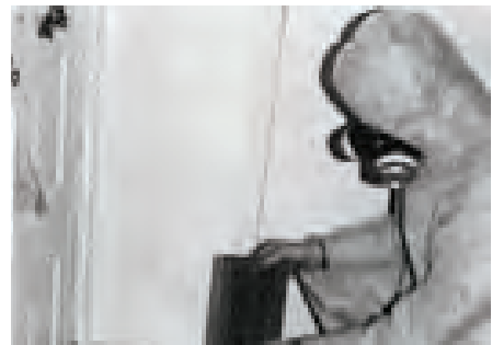
c. Wet wash register covers and replace
