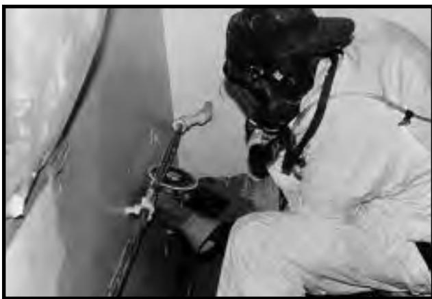
Figure 12.12b Open-Faced Power Sanding or Grinding Is Prohibited.
