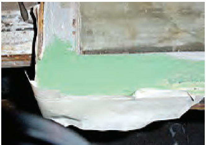
FIGURE 11.10 Rebuild damaged sash with filler or putty.
