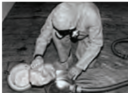
b) Disconnect Vacuum Bag From Hose Inlet
