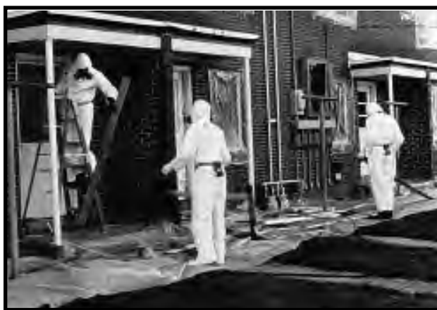
Figure 12.3b Remove and Replace Trim (exterior).
