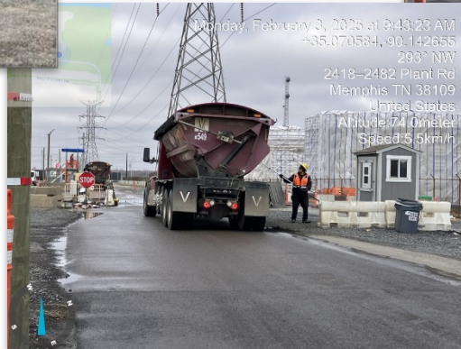
Haul trucks are manually pressure washed prior to the tire wash, a 2 nd tarp observation station and scales prior to leaving the site
