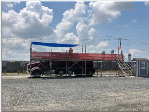
Tarp coverings are inspected prior to staging in loadout area
