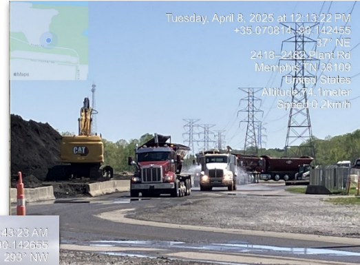
Haul trucks at the loadout area while a water truck maintains dust control
