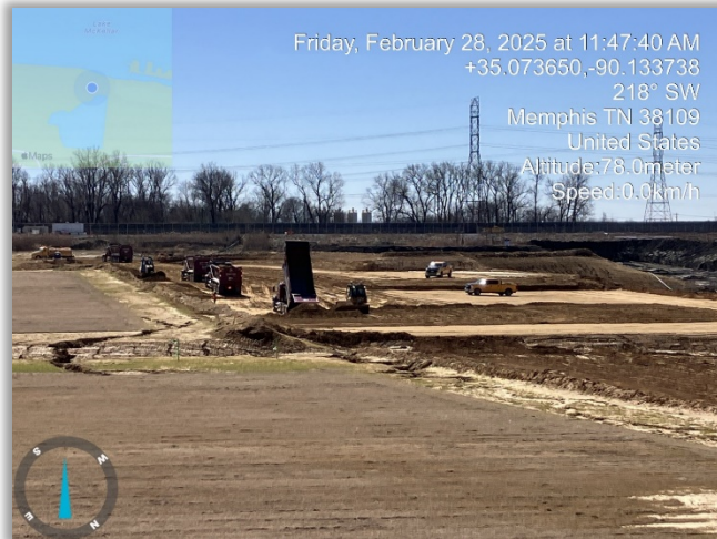
Trucks offloading borrow material along the former stilling pond area
