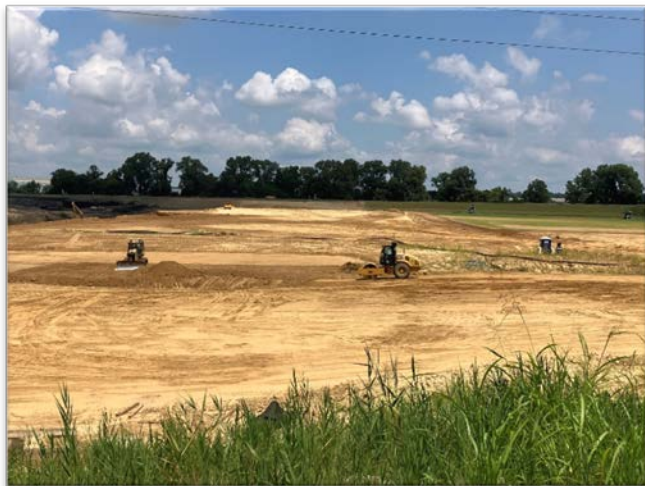
Compacting and grading borrow material
