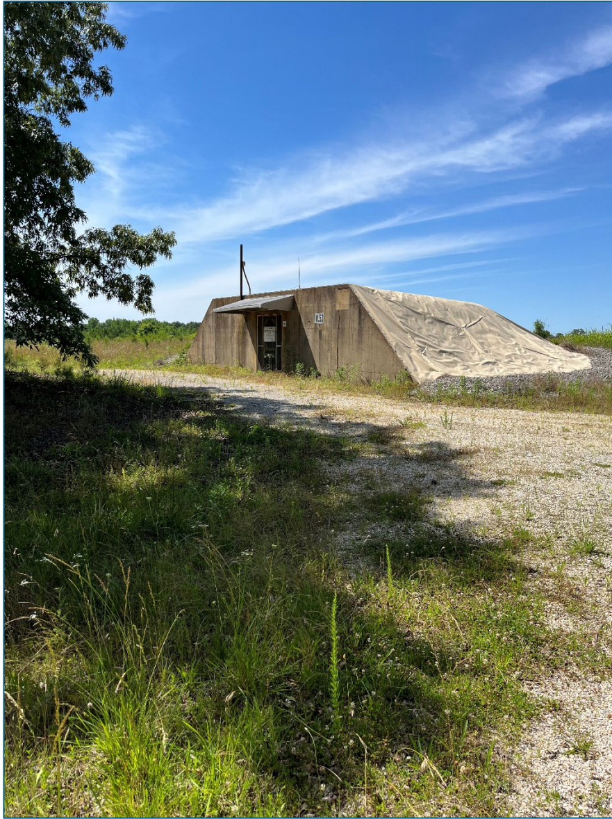
Area W ADA – Building W-53 Shooting Barricade
