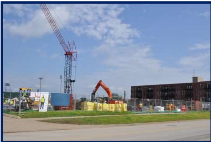
During construction of the state parking garage.
