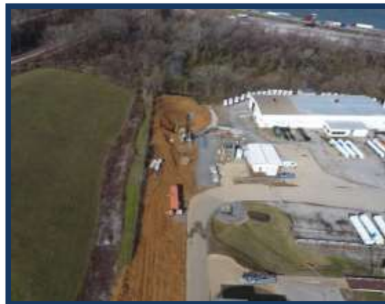
Above, the 10'x10' box culvert. The foundry fill is above native soils. Shortly after this section of the alignment, the foundry fill dramatically increased, along with solid waste and other fill as the sub-surface composition changed throughout the project.
