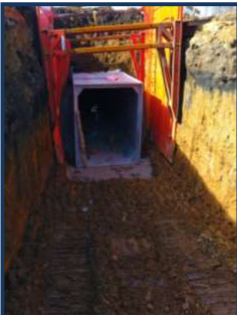
Above, the 10'x10' box culvert. The foundry fill is above native soils. Shortly after this section of the alignment, the foundry fill dramatically increased, along with solid waste and other fill as the sub-surface composition changed throughout the project.
