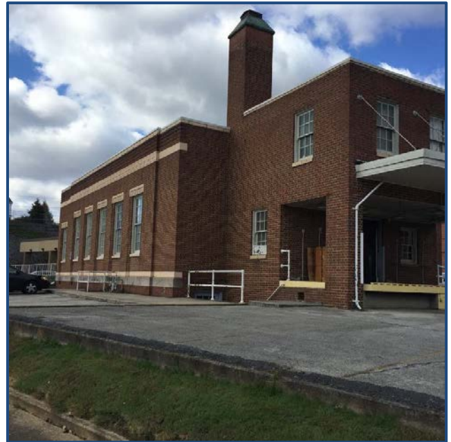
The former post office before new windows were installed.
