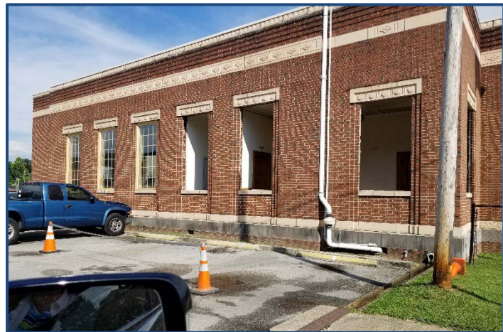
During 2019, the replacement of windows begun.
