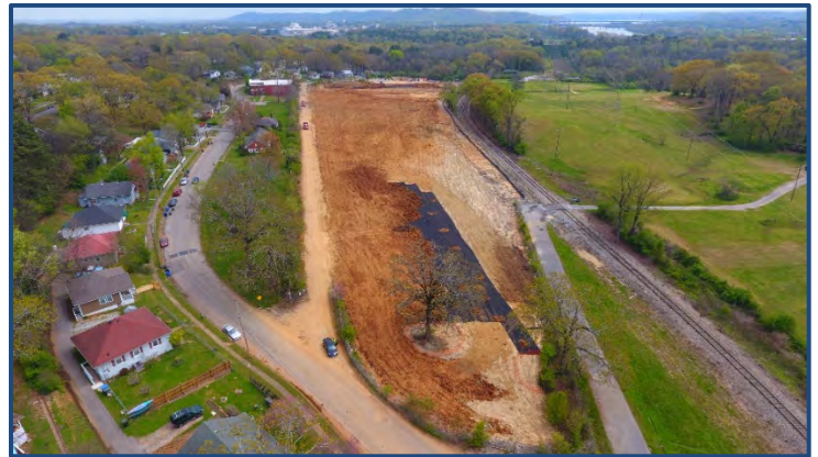
During cleanup of the former Lupton City Mill site hazardous materials were removed and the property was graded and covered.
