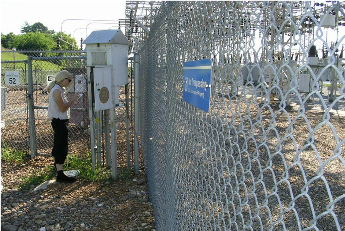
Natalie Pheasant changes air filters at the background station in Loudon County.
