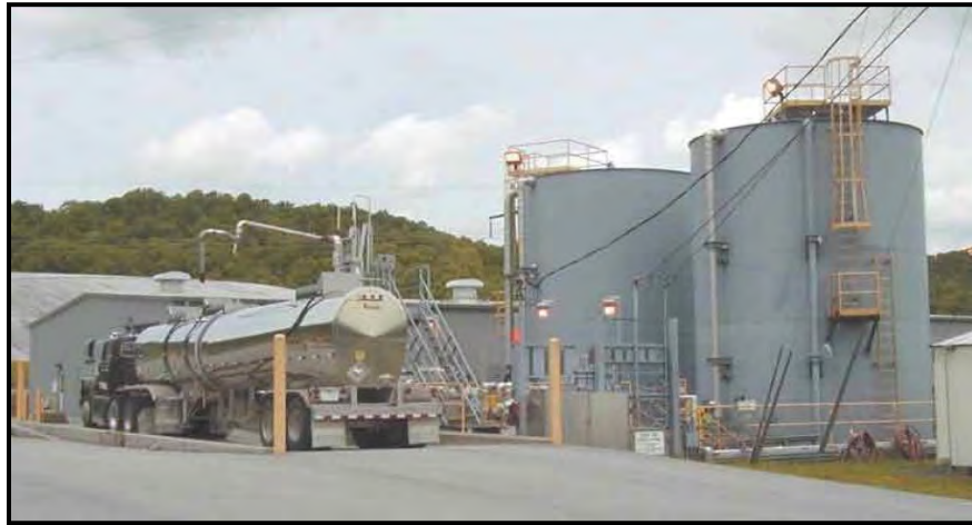
Fig. A.2. Leachate Storage Facility.
