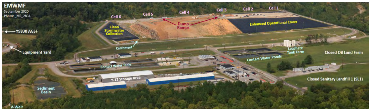
Fig. 3. Environmental Management Waste Management Facility.
