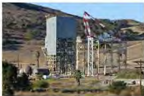
The Sodium Pump Test Facility at the Energy Technology Engineering Center prior to its demolition on Oct. 1, 2021.
