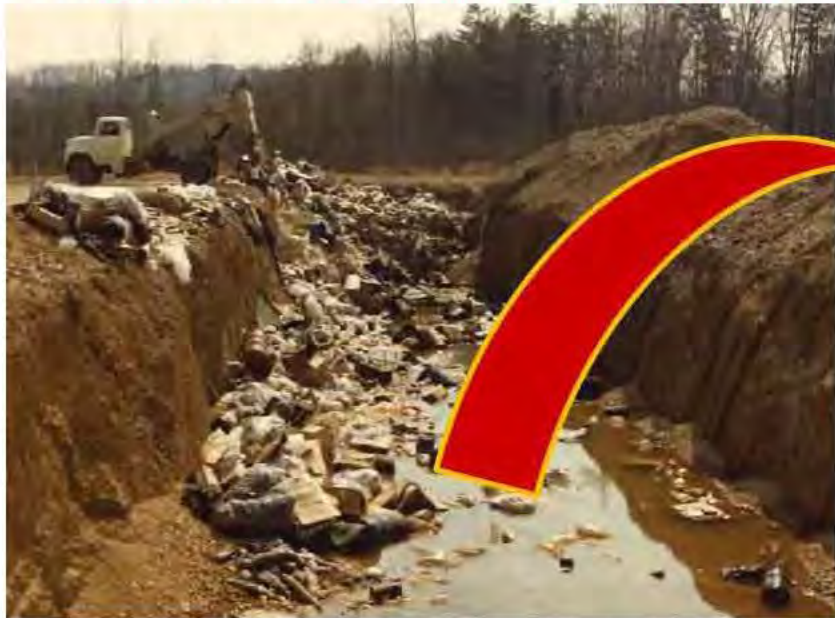
Waste dumped into trenches in Bear Creek Valley prior to DOE establishing requirements for disposal
