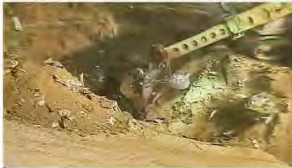
An extended-arm excavator retrieves the final waste from the Accelerated Retrieval Project IX facility on Dec. 6, 2021. The final waste retrieval is pictured on a computer monitor inside a control room at the Idaho National Laboratory Site as access to the retrieval area is controlled for safety.
