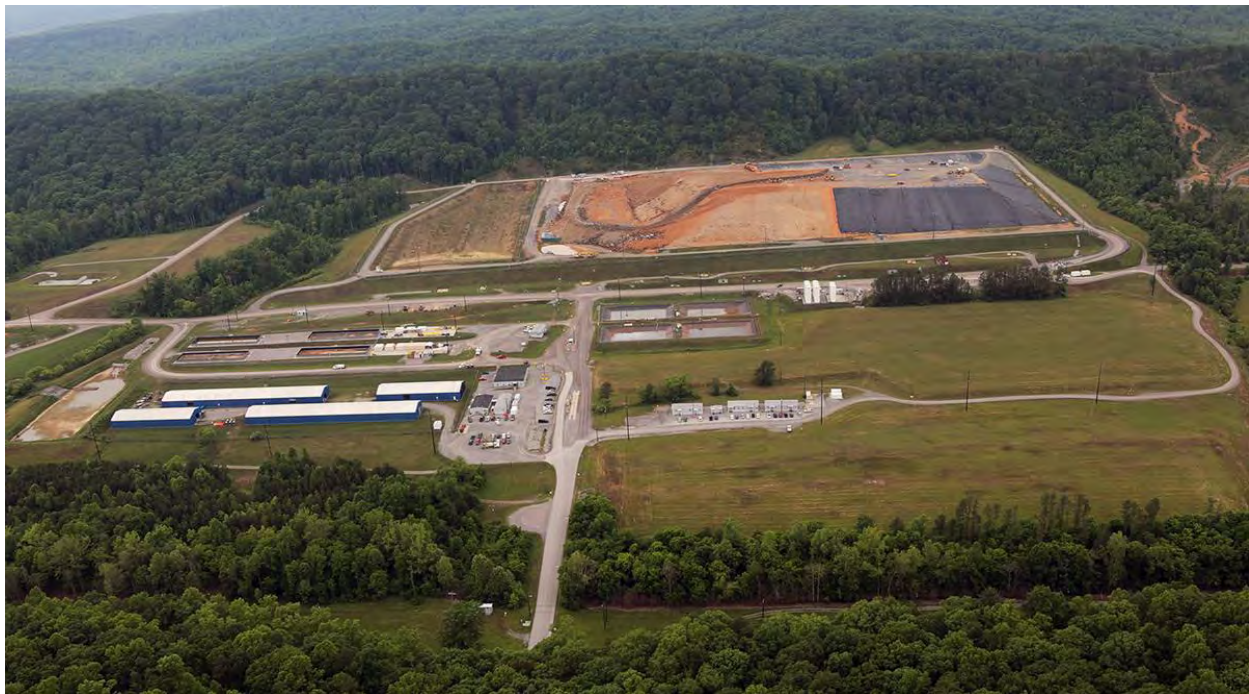
Figure 2. Environmental Management Waste Management Facility.
