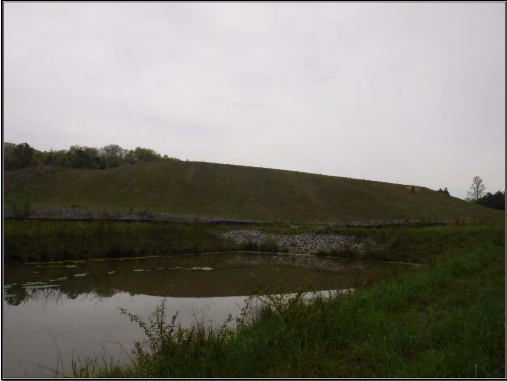
Figure 8. Disturbance and spoil area, facing northeast.
