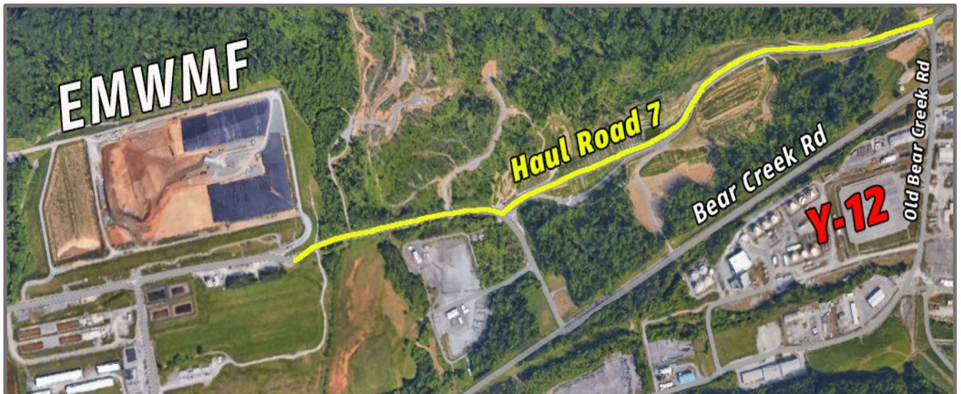
Figure 6.1.4.6: Haul Road Section 7
