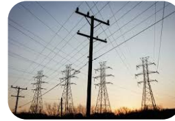
Upgrading Electricity Distribution
