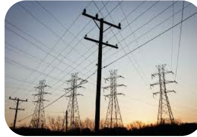
Upgrading Electricity Distribution
