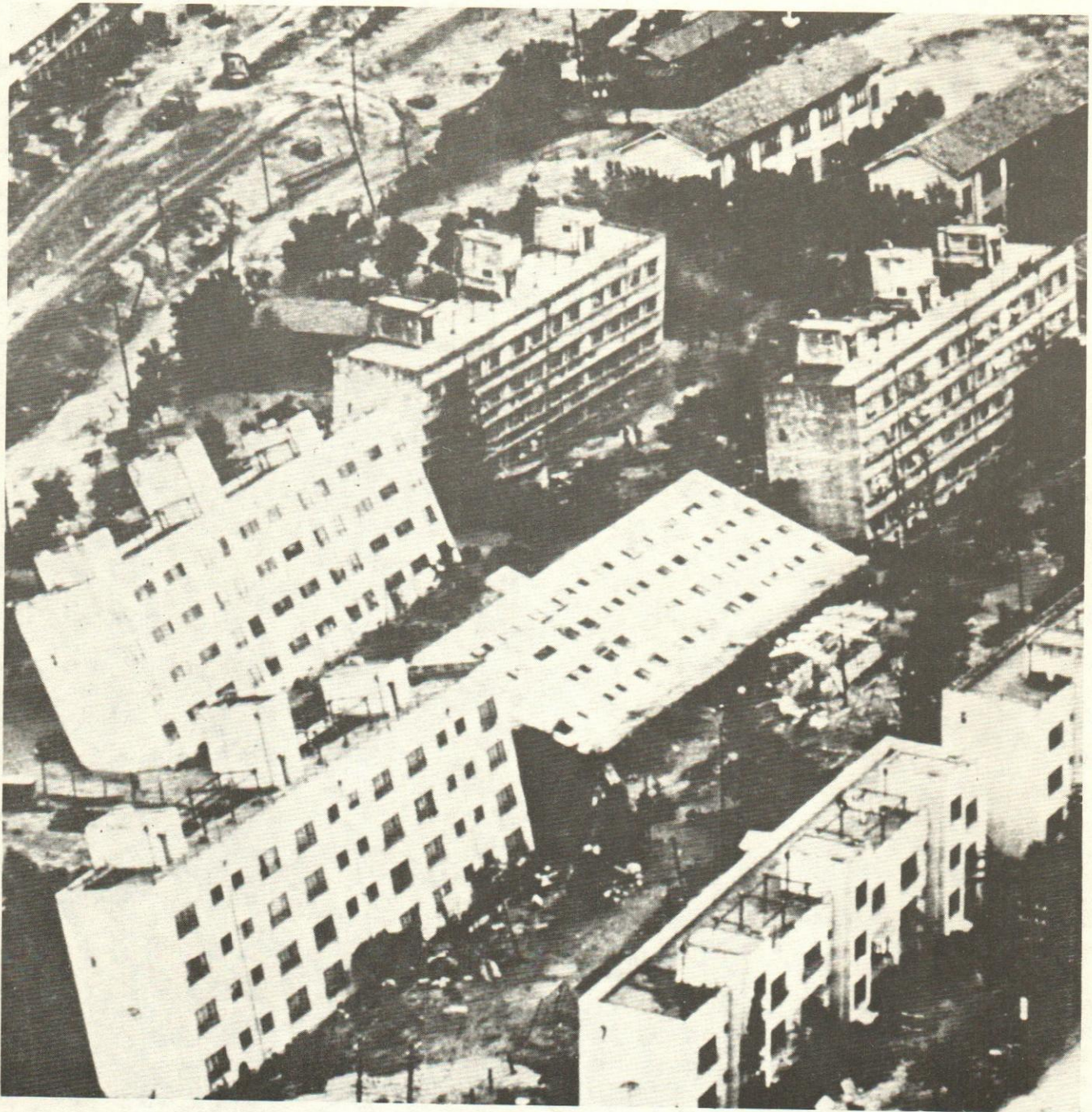
Figure 11. Spectacular effects of soil liquefaction during the earthquake of 1964, Niigata, Japan. Buildings have tipped and sunk into temporarily liquefied earth. Reprinted from U.S. Geological Survey, Earthquake Information Bulletin, v. 8, no. 1, back cover.
